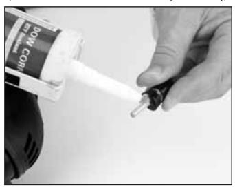
The binding posts are sealed in place with silicone sealant.
