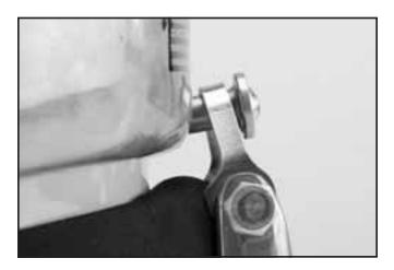
Close-up detail of hinge tab engaging alignment sleeve.
