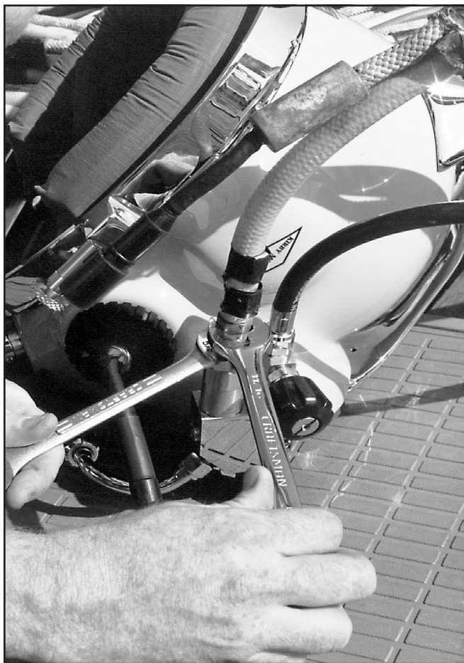
Connecting the umbilical to the helmet.
