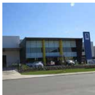
JFD's Training Facility - Bibra Lake, Australia
