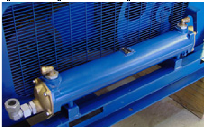
Figure 35 Cooling Water Heat Exchanger Seawater/Freshwater
